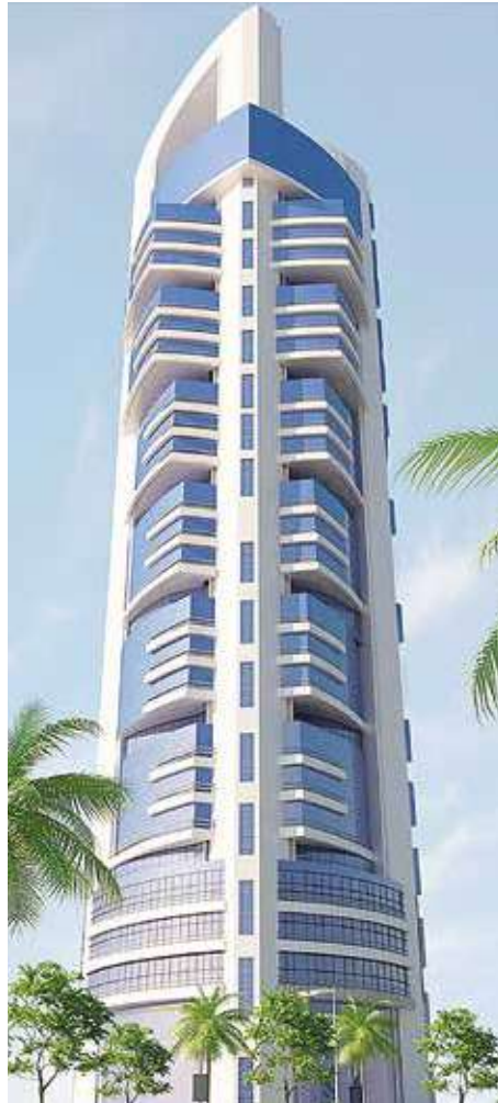
Sylyyah Tower, Qatar
