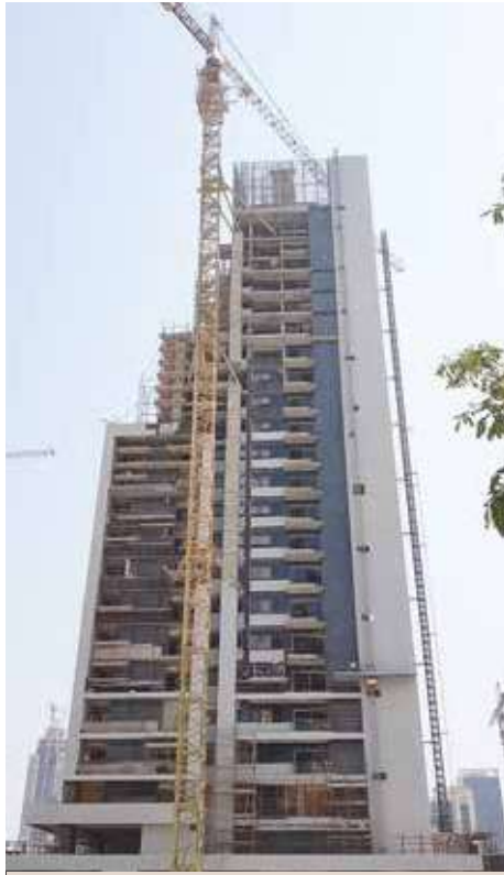
Nuwat Tower, Doha - Qatar
