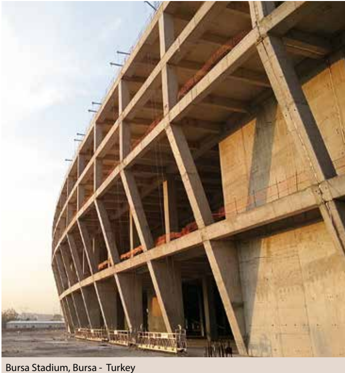
Bursa Stadium, Bursa - Turkey
